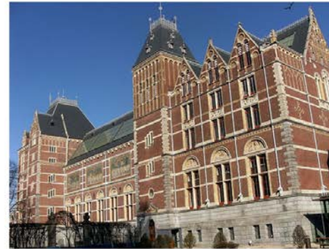
Bricks as building blocks
