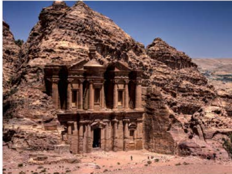
Excavated from solid rock
